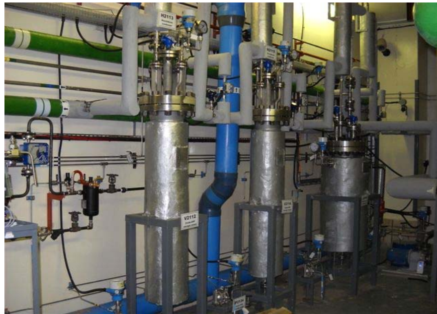
Storage vessels of DF reaction system with utility headers in the background
