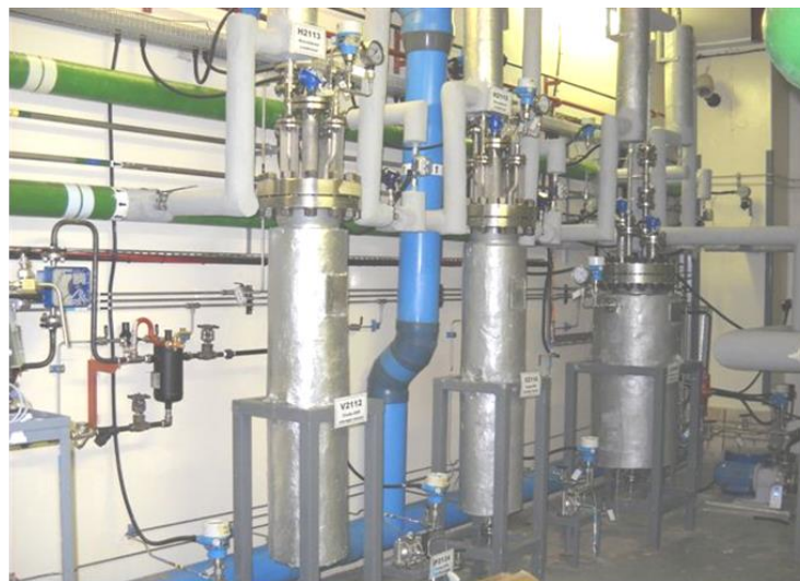
Storage vessels of DF reaction system with utility headers in the background
