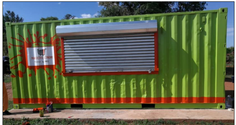
Work has begun in constructing the containers that shall be utilised as retail outlets by qualifying beneficiaries in the Ngaka Modiri Molema District.
