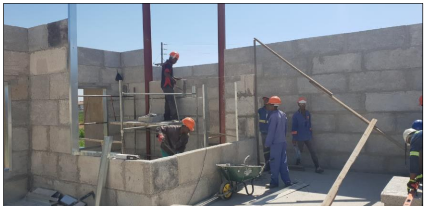
Construction is well-underway in Derby where the NWDC is overseeing the building of a library using alternative building material panels. A second library is being built in Stella.
